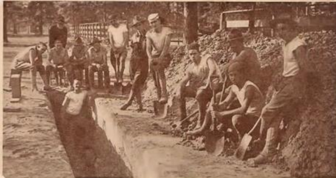
Trench Digging—Camp Logan, Houston, Texas.
