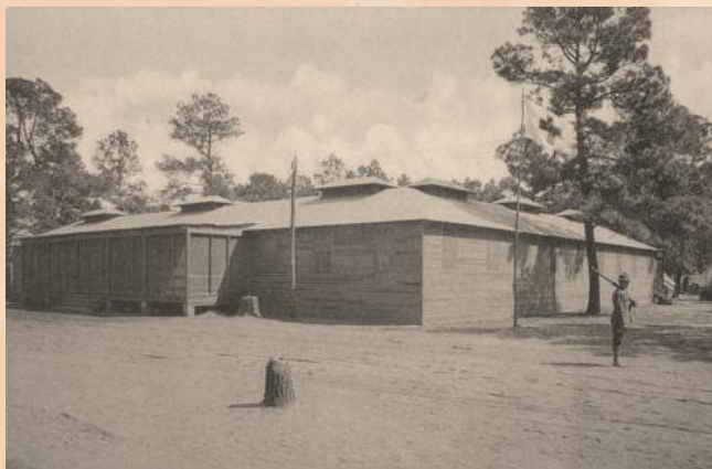
Red Cross Building at Camp Logan
